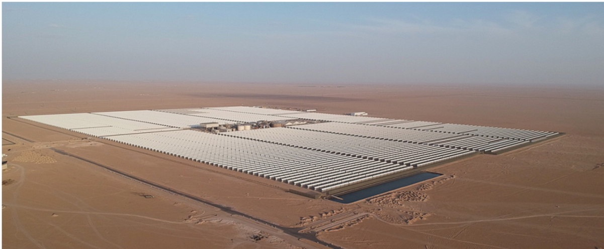
FIGURE 5. Shagaya 50MW CSP Plant
